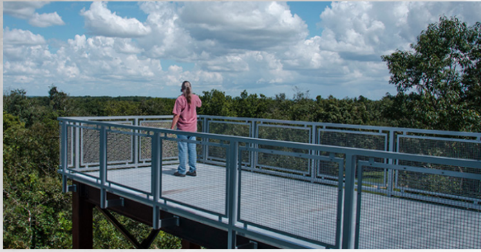
Lookout Tower on Green Mountain Scenic Highway
