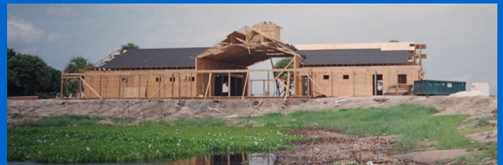
The Lagoon House under construction.
