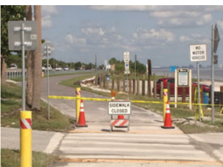
EROSION-RELATED ACTIONS COURTNEY CAMPBELL SCENIC HIGHWAY
